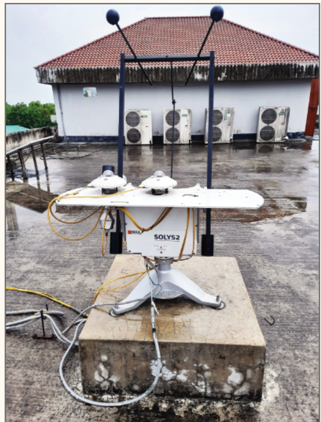
Sun Tracker at PSTU, Patuakhali
